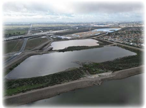
Storm Water Captured in San Sevaime Basins
